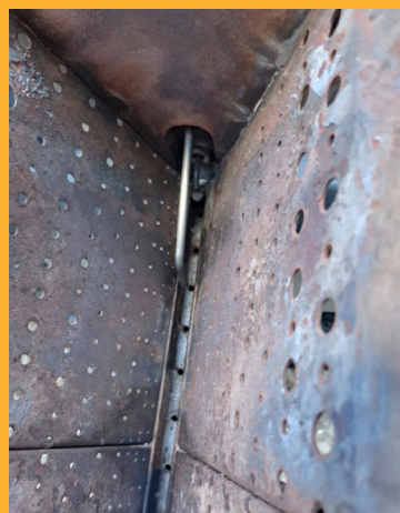
Spark electrode and flame rod unplugged, without debris
